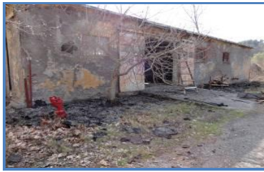
Driving band bldg before
