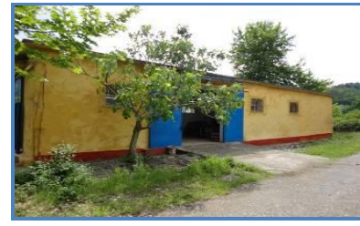
Driving band bldg after refurbishment
