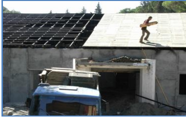
Utilisation of old wooden boxes for refurbishment
